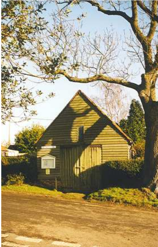
Figure 7 Mature tree by the garage to Wheelwrights
